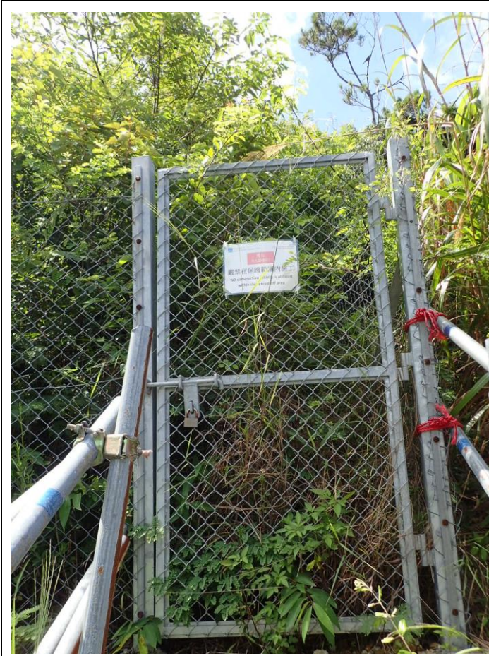
Photo 3 – Current situation of fencing and warning sign
